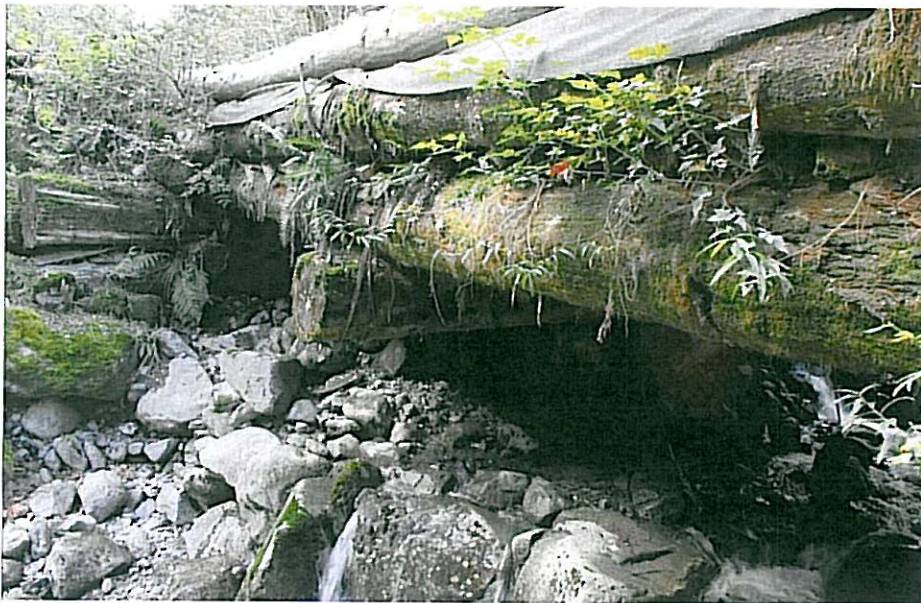
CK-2267 From Downstream
