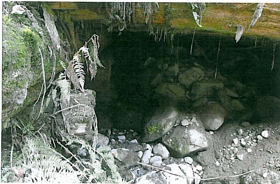
CK-2267 Right Abutment
