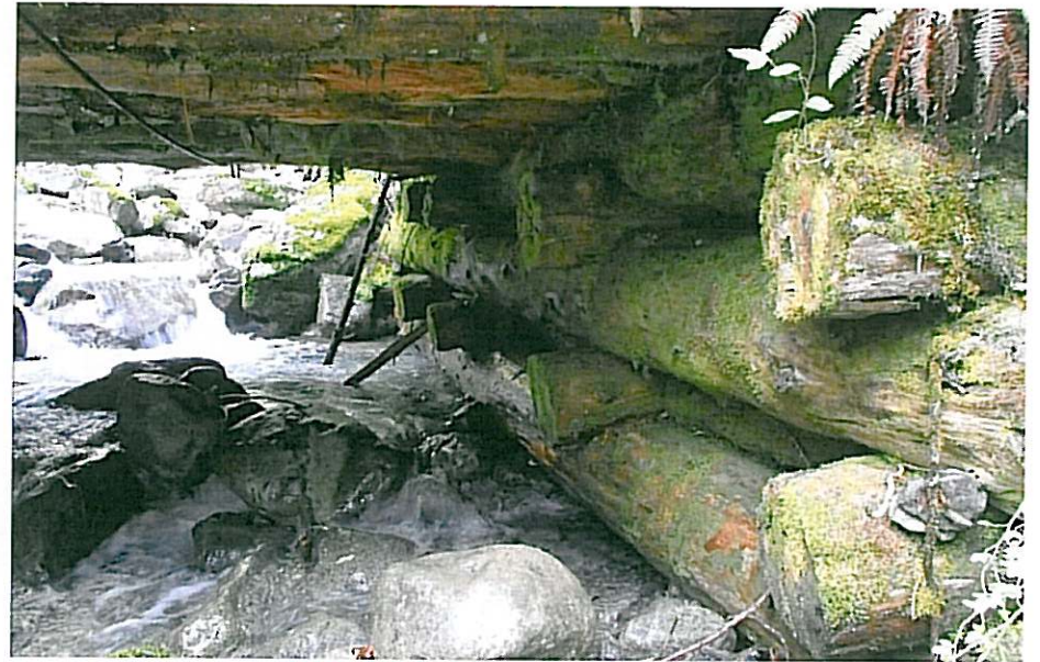
CK-2267 Left Abutment
