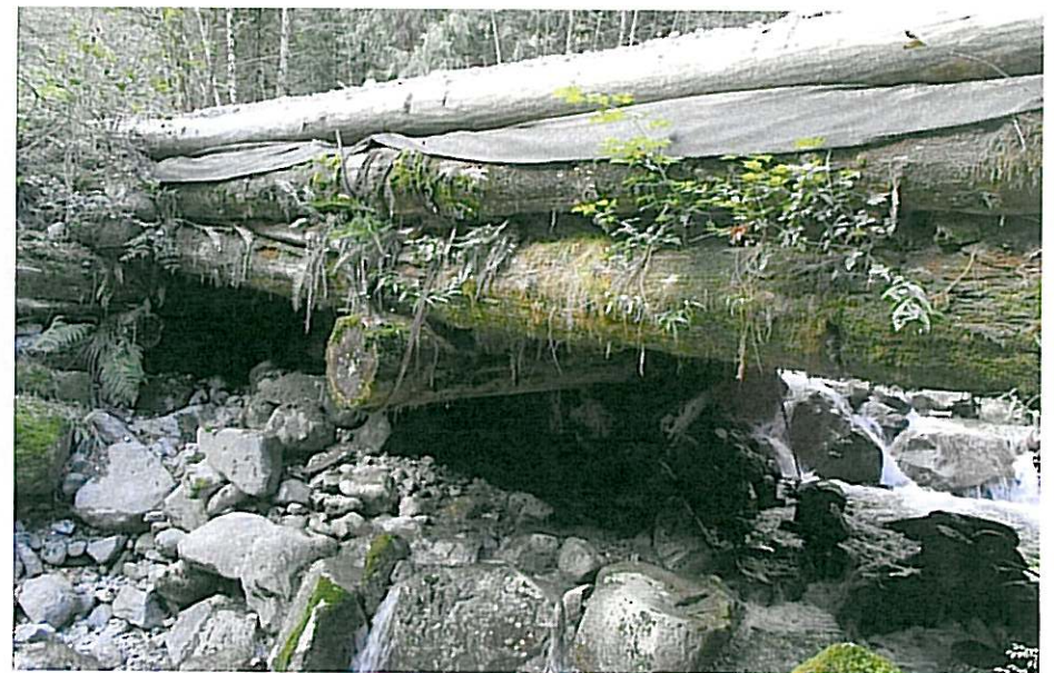
CK-2267 From Downstream (2)
